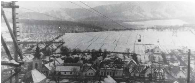
The wire-cableway of the Hungária coal mine above Pilisszentiván
